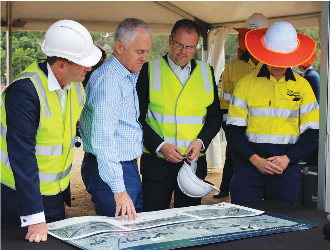
Ted with the Hon Malcolm Turnbull, Prime Minister, inspecting upgrade construction on the Bruce Highway
